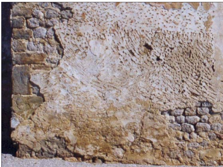
Figure 10: Church of Sts Primus and Felicianus at Gorenje Karteljevo. South wall of the nave; example of stratified composing of stones.
