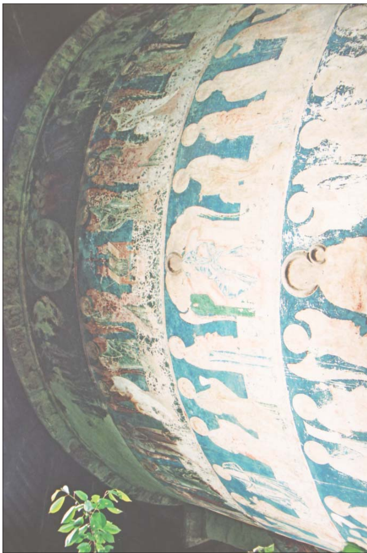
Figure 34: Church of the Beheading of Saint John the Baptist Arbore; southern apse; the surface painted with blue azurite is much better preserved than surfaces in other colors.
