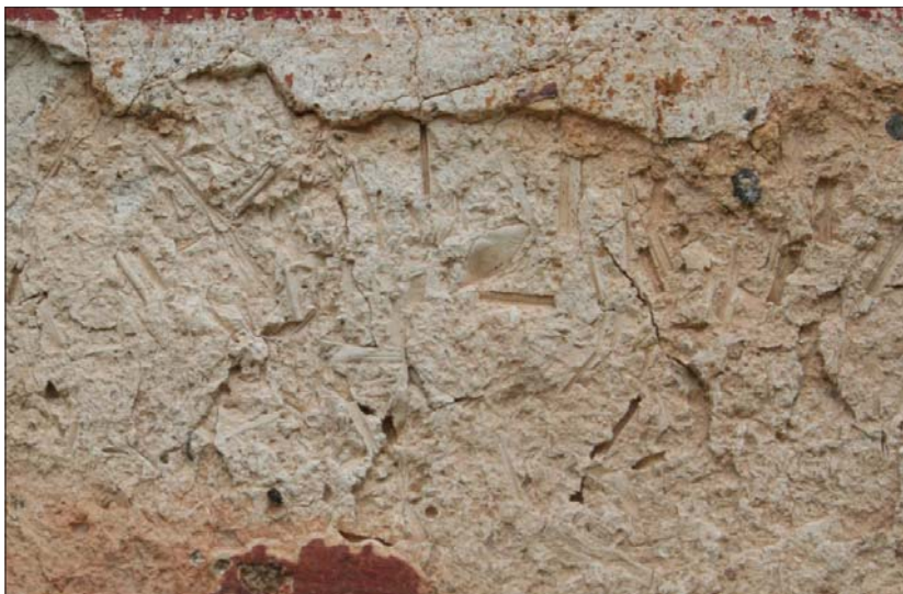
Figure 12: Church of St. Nicholas at Rasca, southern wall; cut straw in the plaster.
