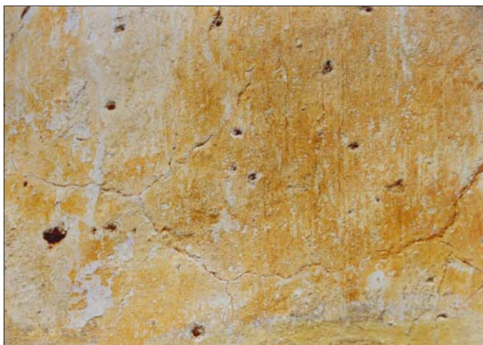
Figure 13: Church of St. Martin at Zalog, southern wall; particles of crushed brick in the plaster that caused damage in the form of eruptions.
