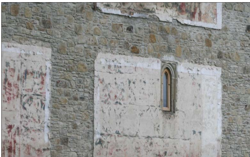
Figure 11: Church of the Dormition of the Virgin at Baia, southern wall; clearly visible masonry where wall paintings were detached.
