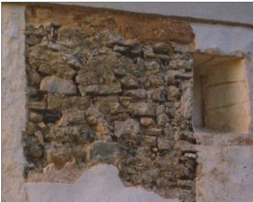
Figure 9: Church of St. Urh at Vihre. South wall of the nave; example of irregular composing of stones.
