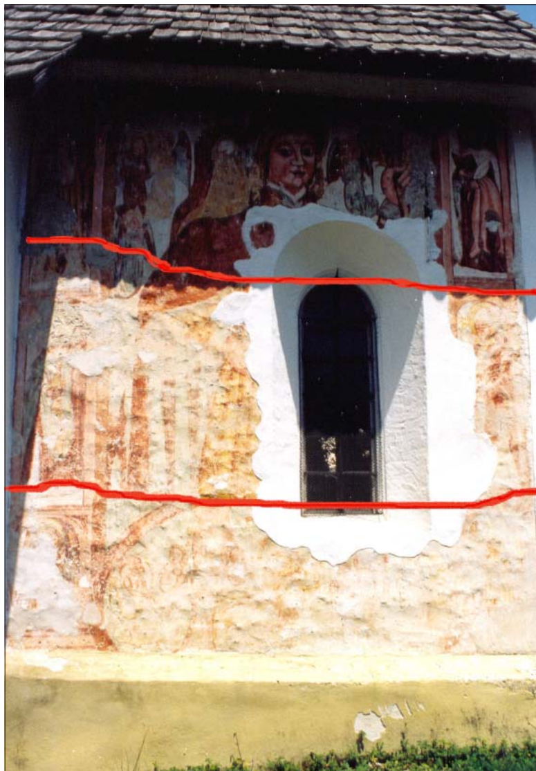
Figure 24: Church of Mary Magdalene at Brod in Bohinj, southern side of the presbytery; the lowest section of the painting is marked by combined influence of capillary action of ground moisture and precipitation.
