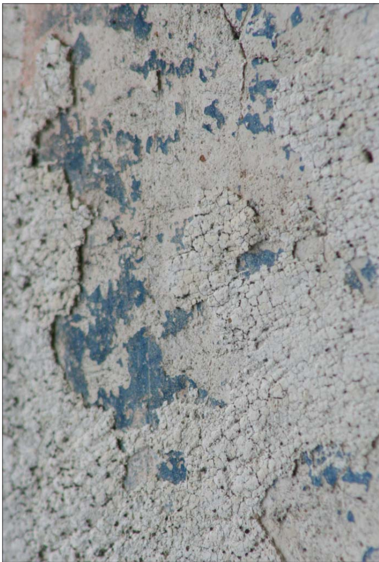
Figure 29: Church of the Feast of the Annunciation at Moldovita, northern wall; thick whitewash or very thin plaster that covered the remnants of original painting also flaking off the wall.
