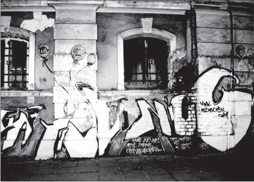
Illustration 3: Nd2Nd. Legal Piece on the Facade of a Public Building. Photo Miglena Ivanova, 2004.
