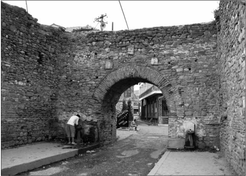
Fig. 2. Elbasan, Albania. Southern or bazaar gate, exterior: the three blocks of white marble quoted by Evliya Çelebi.
